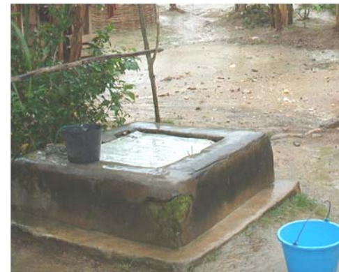
School well. (shallow hand-dug; note cover and lock)
