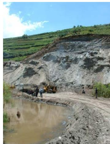
**Excavation of roadbed material from hillside for cross-wetland traverse**
